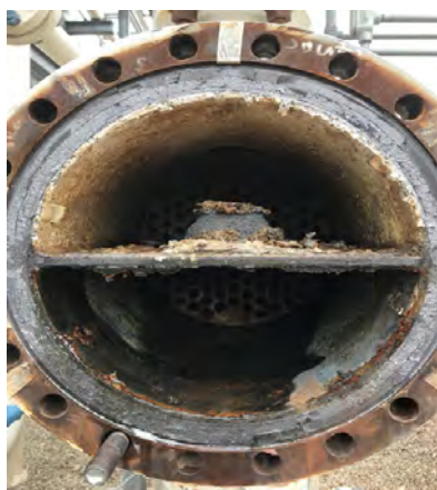
South Side of HEX Before & After Cleaning
