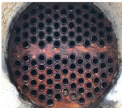
North Side of HEX Before & After Cleaning
